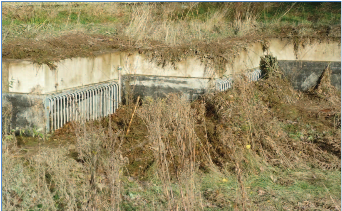
Plate 5 - Ruthin Link Road Culverts (Post November 2012 Flooding)
