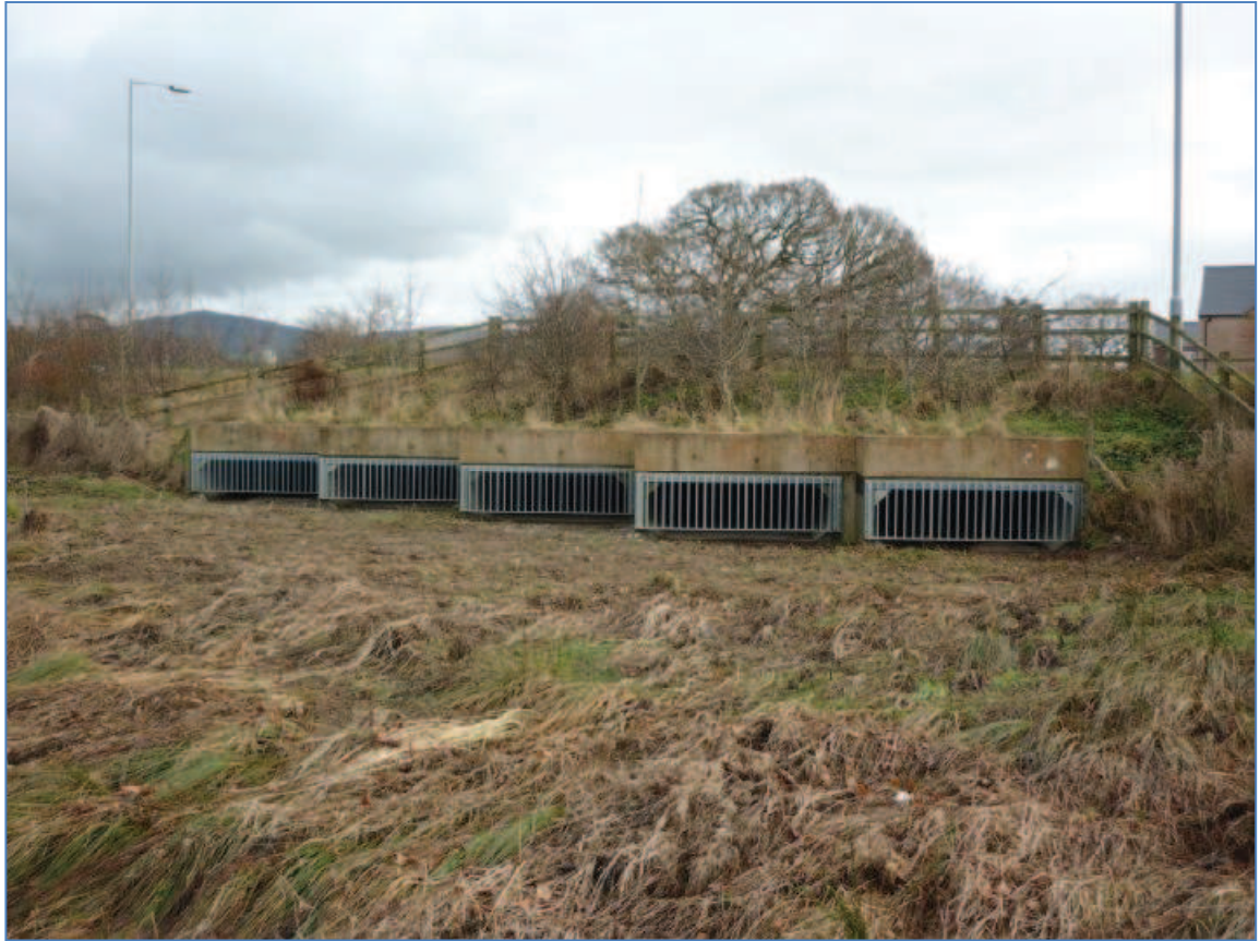
Plate 4 - Ruthin Link Road Culverts
