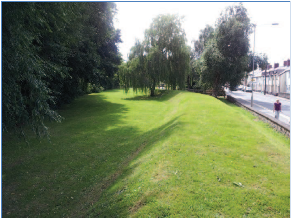
Plate 6 - Ruthin Flood Embankment adjacent to Park Road: Constructed in 2003
