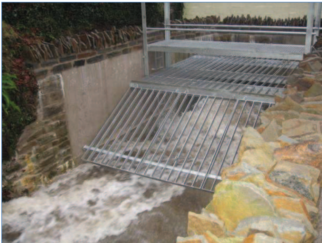
Plate 13 - Typical Raking Screen, Cwmfelinfach, Caerphilly
